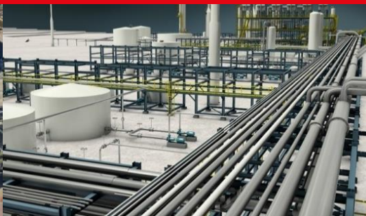
Pipe Racks 75,892 tons
