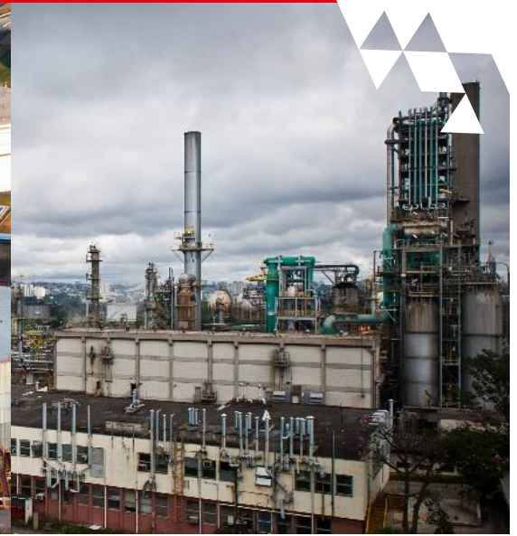
Construction of Chemical and Petrochemical Plants
