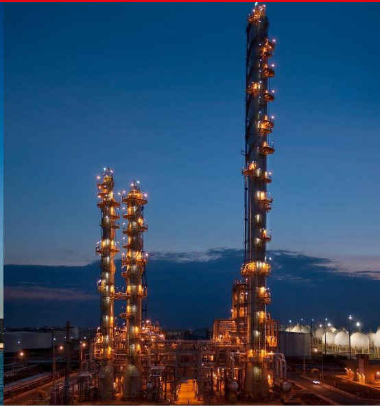
Construction of Refineries
