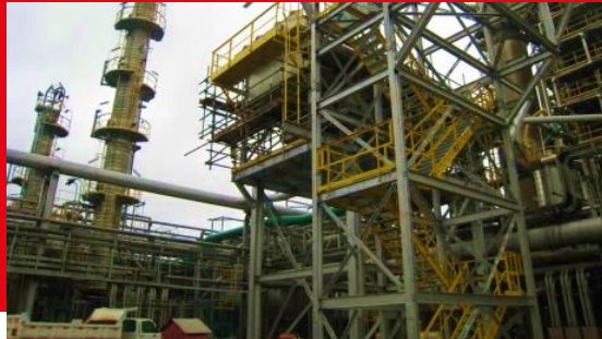
Metallic Structure 564,157 tons
