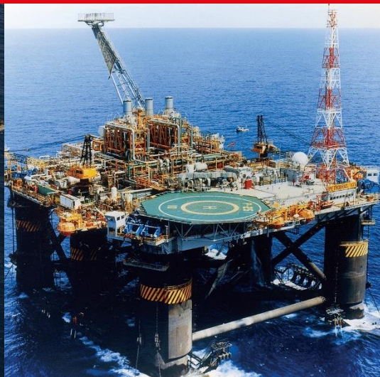
(SS) P-25 , 1996 Conversion of Semi-Submersible Drilling Unit into a Semi-Submersible Production Unit, with a process plant of 100,000 bopd and 115 mmcf/d of natural gas.
